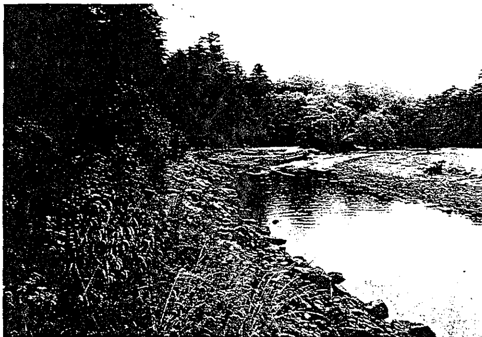
Figure 3.8. Indian River bank protected with riprap to prevent bank erosion. This fill creates an artificial stratigraphic profile along the river bank.
