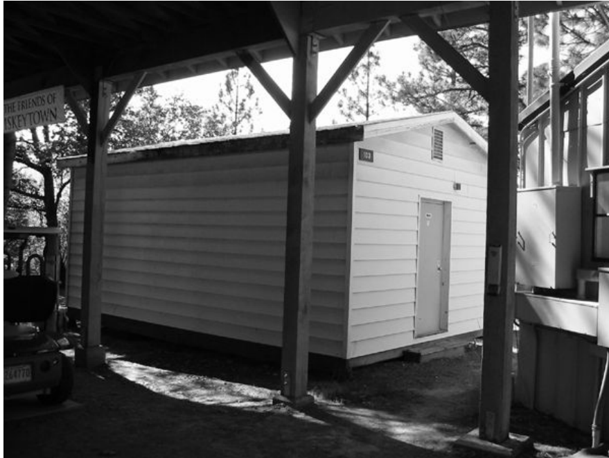
Figure 2 Bally Building at WHIS. Collections removed from this building were taken to REDW SOC museum storage area in 2005.
