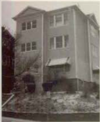
Triple-decker mill housing is found throughout the Valley. Poor renovations eliminate character.
