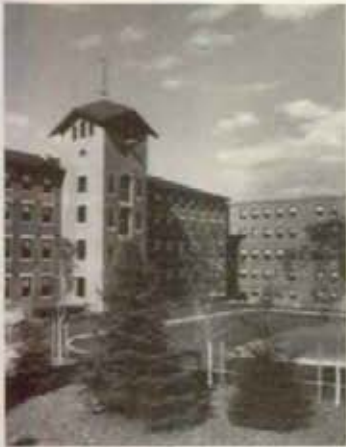
Housing is often the best adaptive reuse for old mills; all are not suitable for modern industry. This mill, formerly the Valley Falls Mill in Central Falls and built in 1849, was adapted in 1979.
