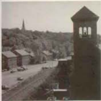
Ashton, RI. "If you lived here during the last century, your whole day, and much of your life would have been confined to the 1/4 mile distance between the mill and the edges of the village. Most workers had only to walk about 200 feet from their doorstep to the factory."
