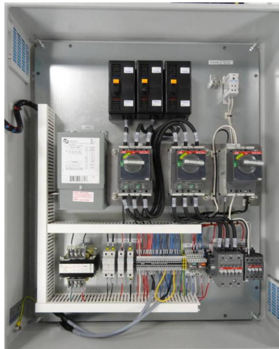
Figure 3 Nova NEAVWB80AVWB MDP- Inside
