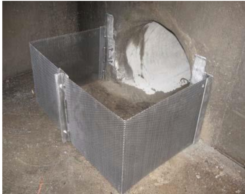
Figure 5-8. Trash Capture Screen
