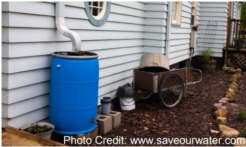
Image 1. Example Rain Barrel at Downspout
