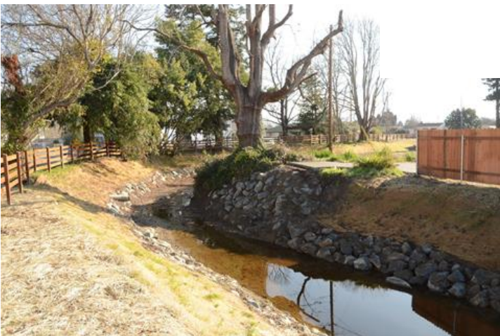
Image 16. Example Rock Slope Protection and Detail.
