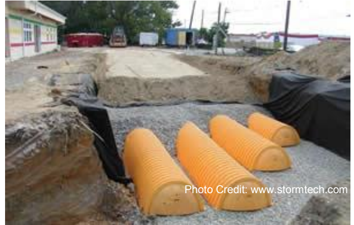
Image 8. Example Sub-surface Detention System
