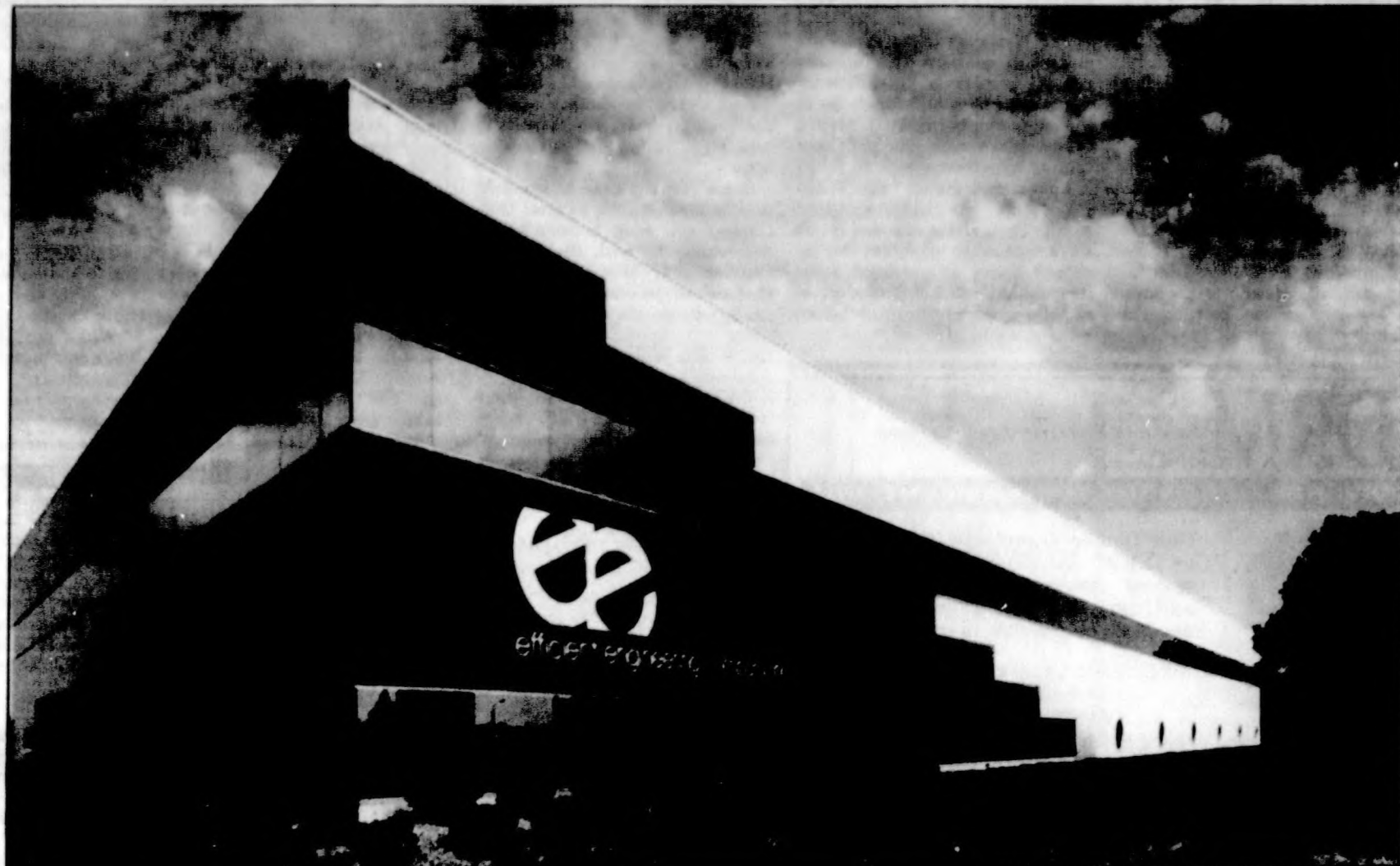
Creative mix: Red porcelain enamel panels blended with precast concrete and glass make for an impressive appearance at this building in Troy.
