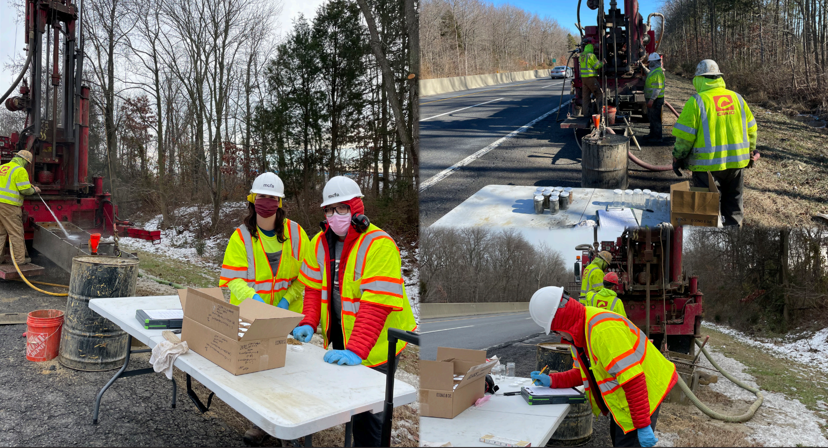
New Jersey Turnpike Authority (NJTA) 1-4 Widening Program, New Jersey
