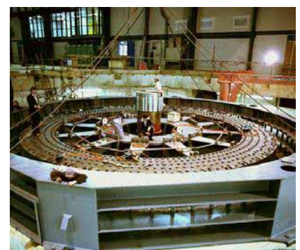
Figure 26.15. One of the two flywheels at the fusion research facility in Culham, under construction. Photo: EFDA-JET. www.jet.efda.org .
