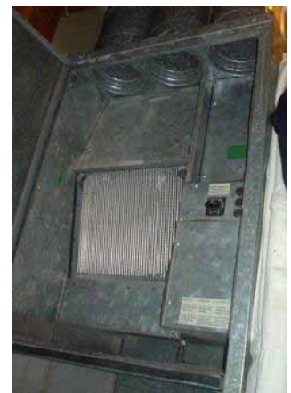
Figure E.11. The Heatkeeper's heat-exchanger.
