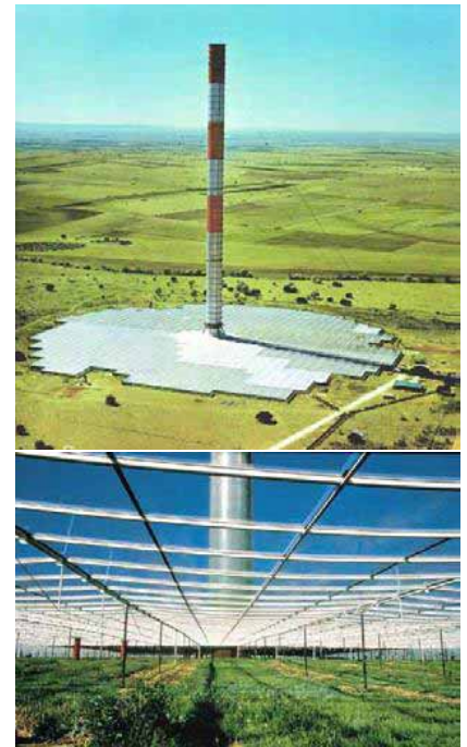
Figure 25.10. The Manzanares prototype solar chimney. Photos from solarmillennium.de .
