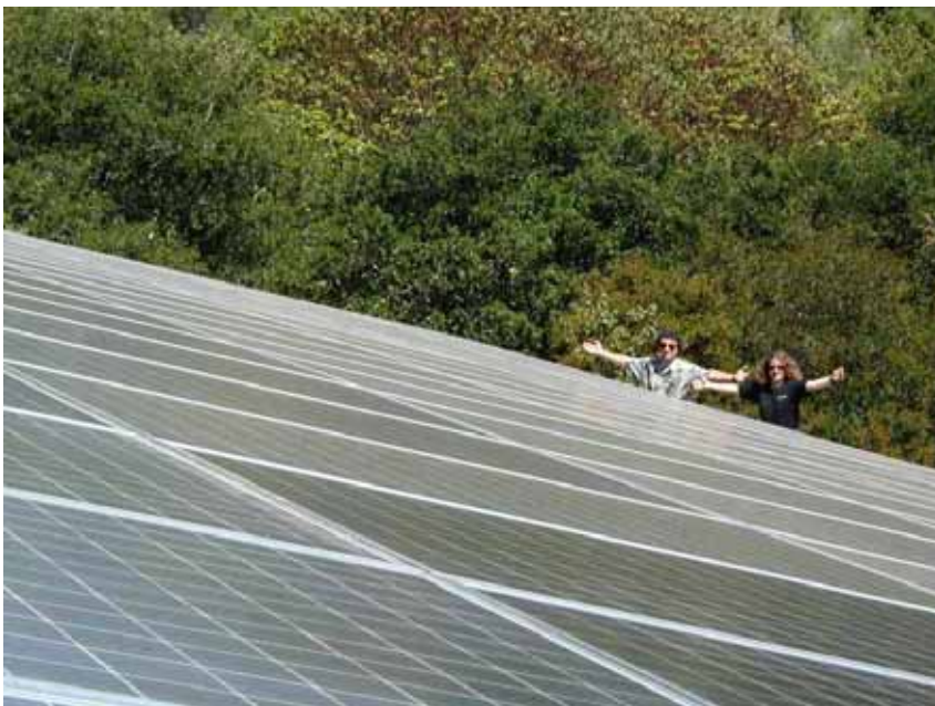
Figure 6.6. Two solar warriors enjoying their photovoltaic system, which powers their electric cars and home. The array of 120 panels (300 W each, 2.2\text{ m}^2 each) has an area of 268\text{ m}^2 , a peak output (allowing for losses in DC-to-AC conversion) of 30.5 kW, and an average output – in California, near Santa Cruz – of 5 kW ( 19\text{ W/m}^2 ). Photo kindly provided by Kenneth Adelman. www.solarwarrior.com
