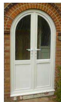
Figure 21.6. A new front door.
