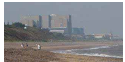
Figure 24.9. Sizewell's power stations. Sizewell A, in the foreground, had a capacity of 420 MW, and was shut down at the end of 2006. Sizewell B, behind, has a capacity of 1.2 GW. Photo by William Connolley.
