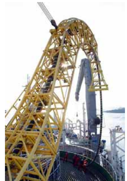
Figure 25.7. Laying a high-voltage DC link between Finland and Estonia. A pair of these cables transmit a power of 350 MW. Photo: ABB.
