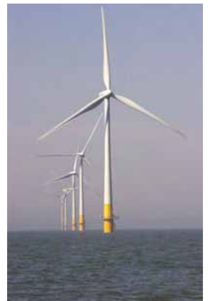
Figure 10.1. Kentish Flats – a shallow offshore wind farm. Each rotor has a diameter of 90 m centred on a hub height of 70 m. Each “3 MW” turbine weighs 500 tons, half of which is its foundation. Photos © Elsam ( elsam.com ). Used with permission.
