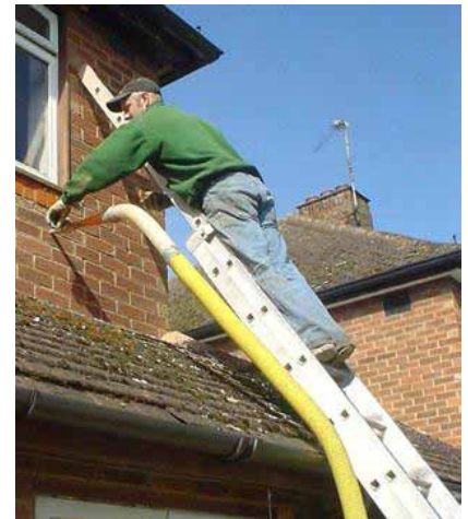
Figure 21.5. Cavity-wall insulation going in.
