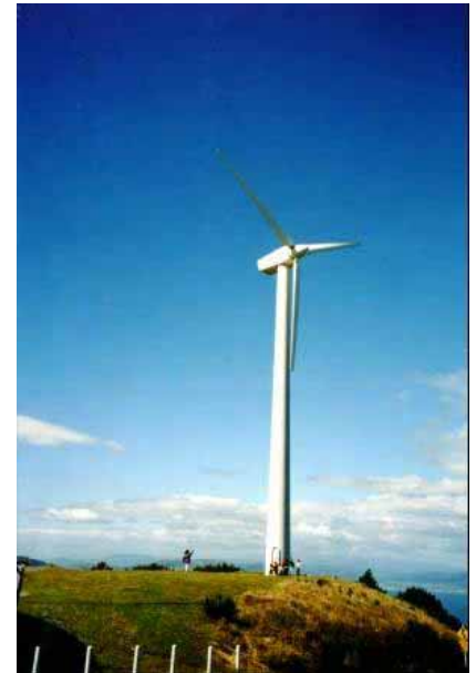
Figure B.3. The Brooklyn windmill above Wellington, New Zealand, with people providing a scale at the base. On a breezy day, this windmill was producing 60 kW, (1400 kWh per day). Photo by Philip Banks.
