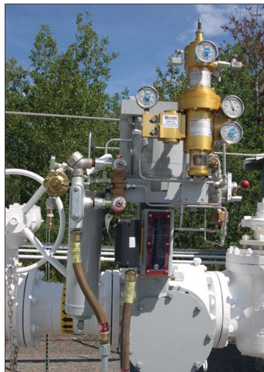
Figure 9 - Model VRP-B-CH with Electrical Override
