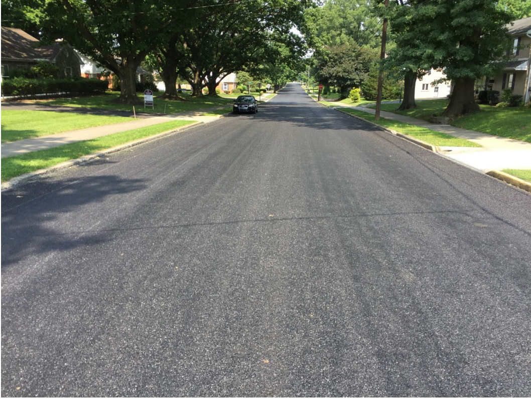
Figure 3: Final seal coat for N. Penn Street.
