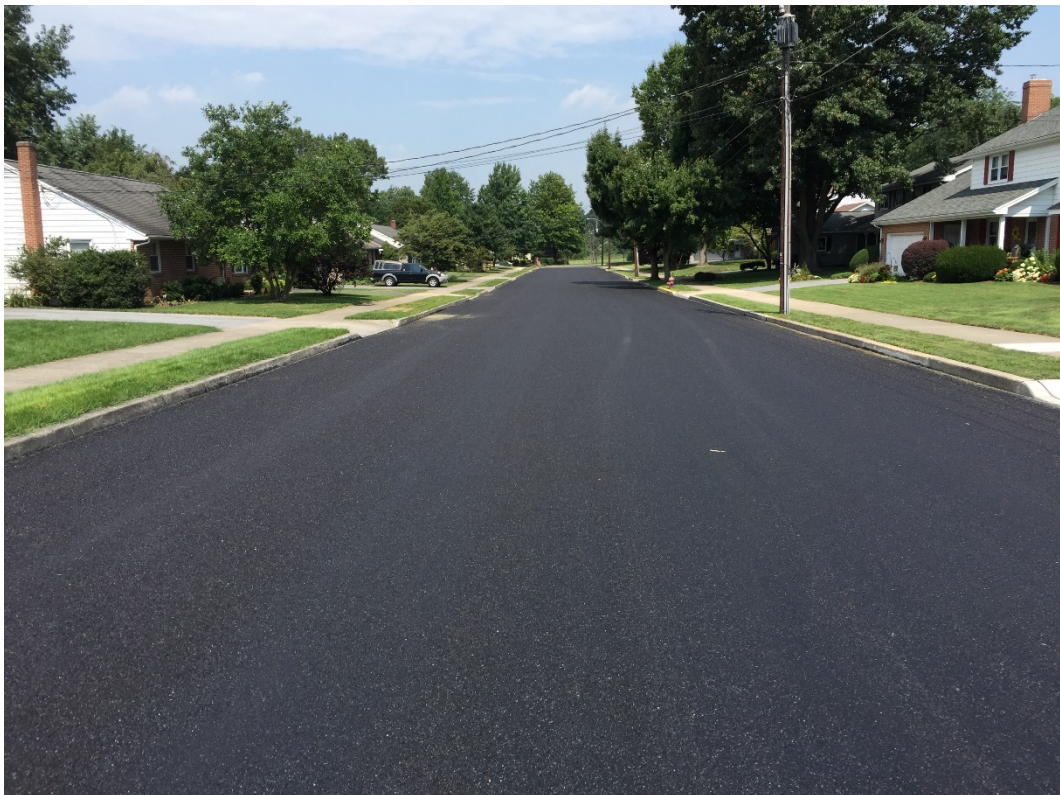
Figure 2: Final seal coat for N. Fulton Street.
