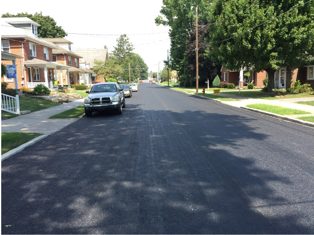
Figure 1: Final seal coat for S. Linden Street.
