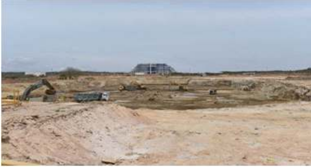
Excavation for KKNPP Unit-4 Reactor Building and Turbine Building under progress
