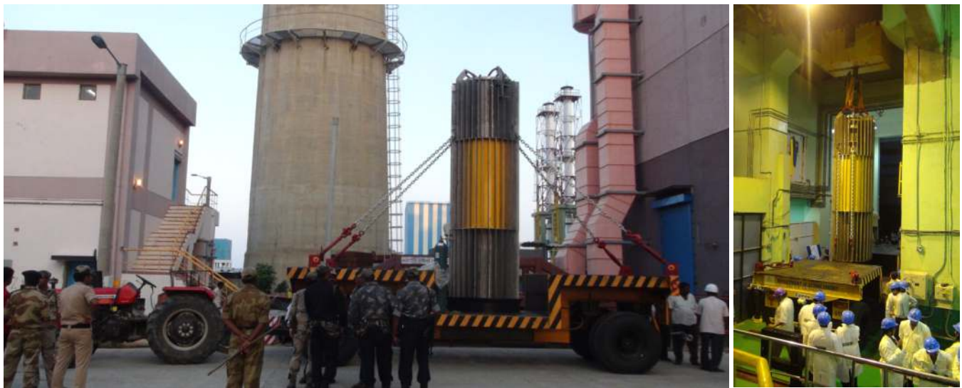
Pre-Commissioning activities in progress at PFBR site
