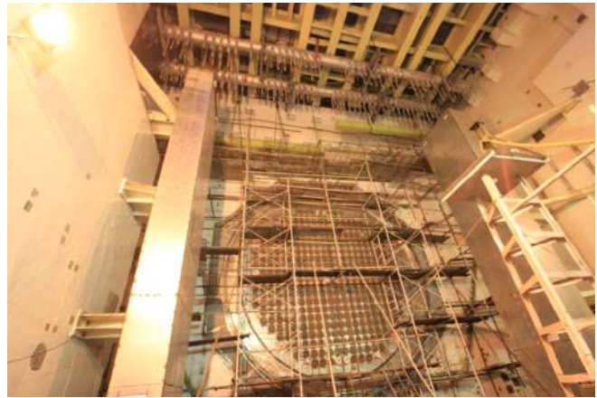
Erection activity in progress at the reactor building of RAPP- 7 & 8
