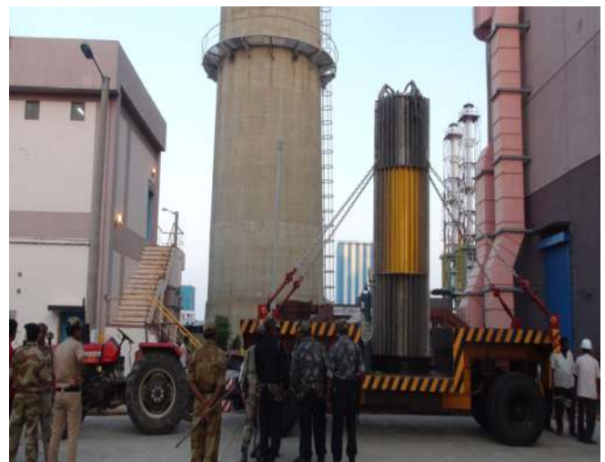
Pre-Commissioning Activities in progress at PFBR Site,
