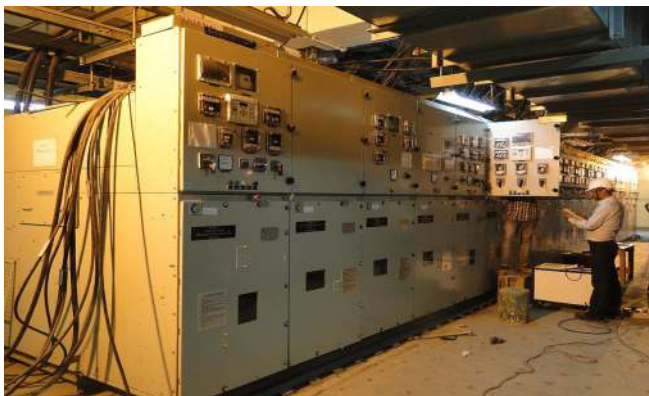
Electrical Installation work in progress at KAPP-3&4
