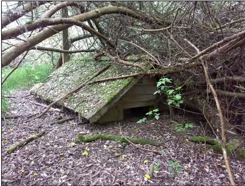
Figure 19. Buried outbuilding on south side of Williams Creek upstream of WCG-1.
