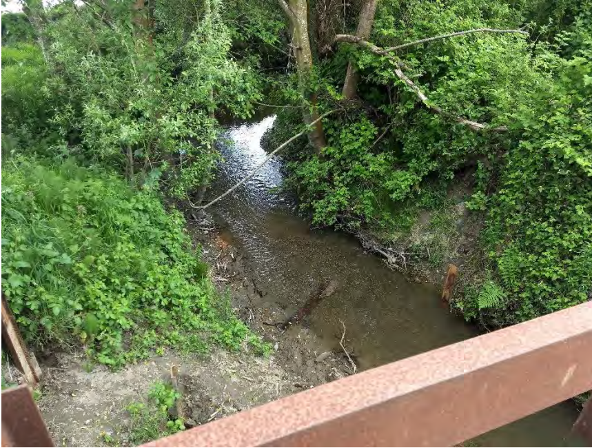
Figure 2-11. Williams Creek in the upper alluvial fan reach. The channel is generally trapezoidal in shape and over 6 feet deep (Photo 2018).
