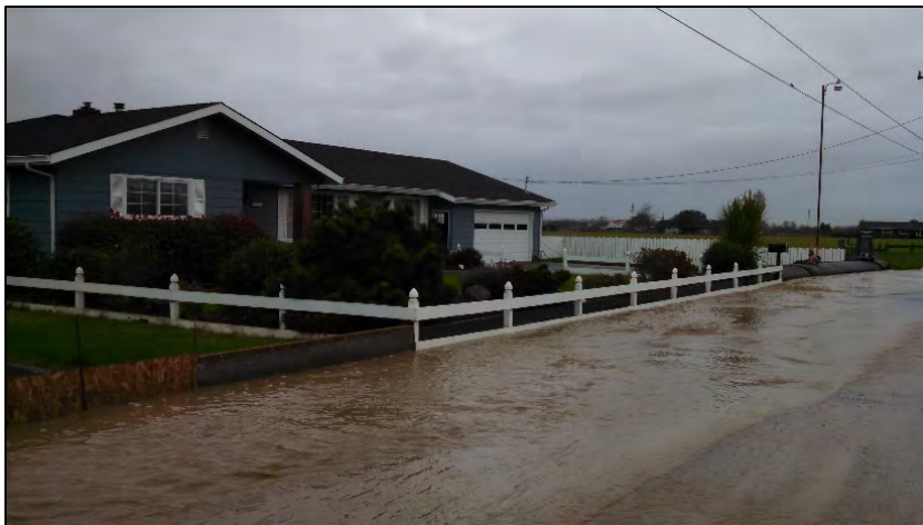
Figure 16. Overbank flows from Williams Creek flowing northward along Ambrosini Lane. Residents have installed various measures for flood protection (Svelha, December, 2015).
