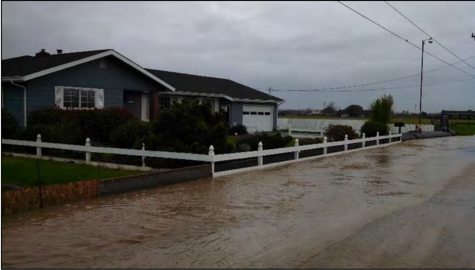
Figure 2-13. Overbank flows from Williams Creek flowing northward along Ambrosini Lane. Residents have installed various measures for flood protection (J. Svehla, December 2015).
