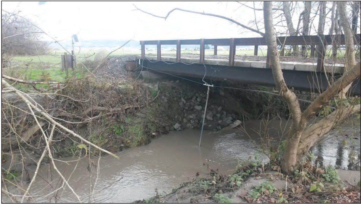
Figure 2. Upstream view of sampling section, turbidimeter boom on cable, gage house and solar panel.
