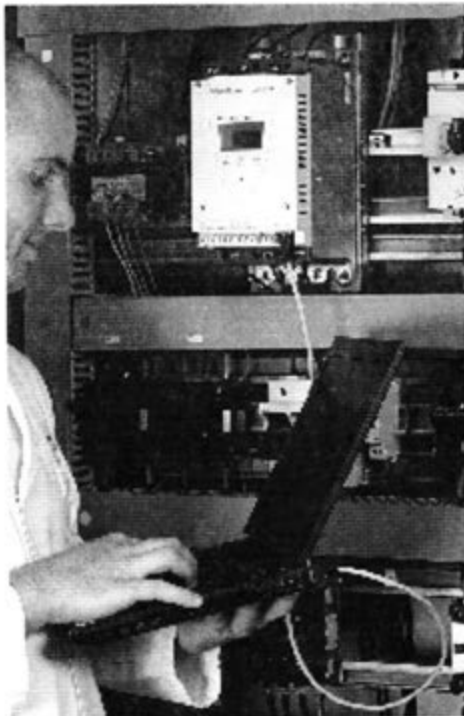
Commissioning the ATS 22 soft start - soft stop unit with SoMove lite setup software
