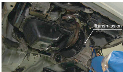
⑩ Reinstalling the Transmission
