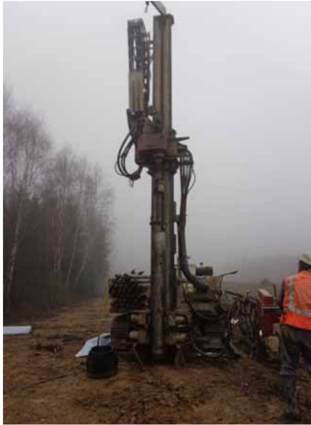
Photo 1 - Machine de forage
