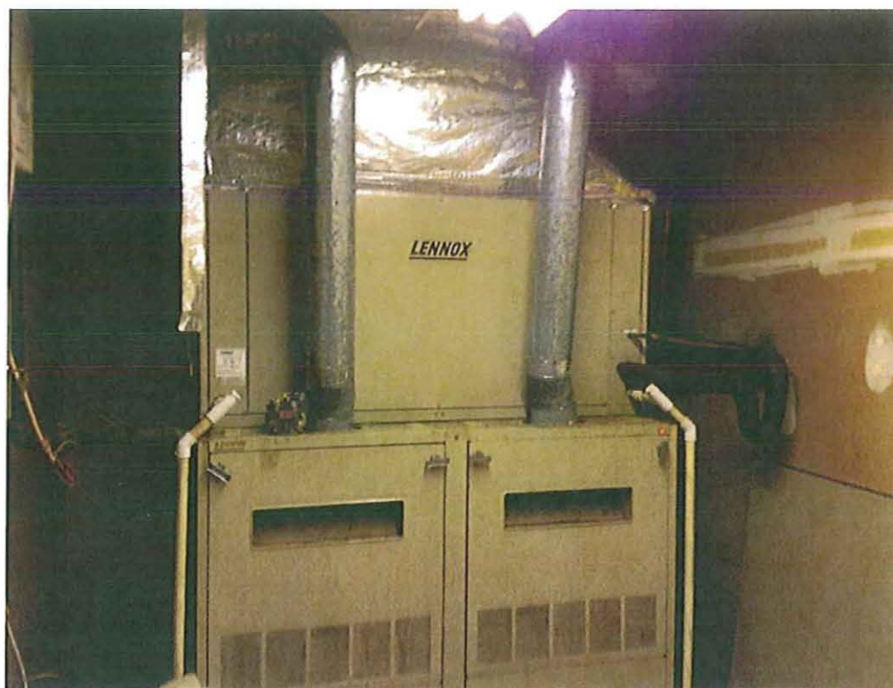
Natural Gas HVAC Unit in Building Interior
