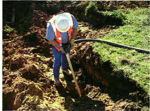
Removal of liquid waste from UST
