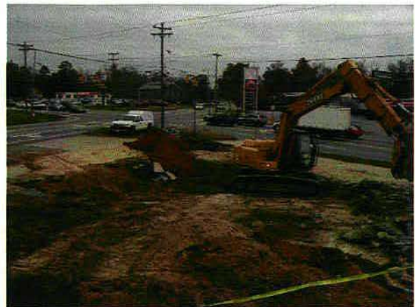
View of site and intersection during site restoration
