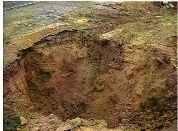
Portion of common tankhold area for UST1 and UST2
