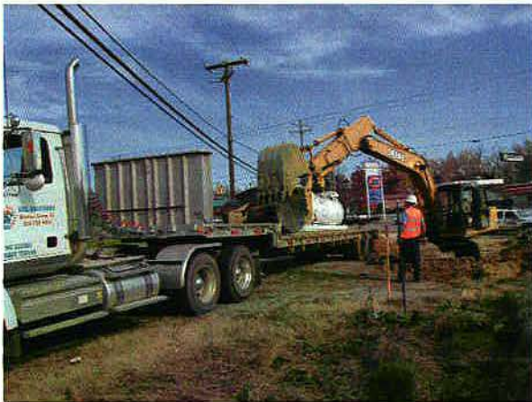
Loading of UST onto flatbed trailer for transport
