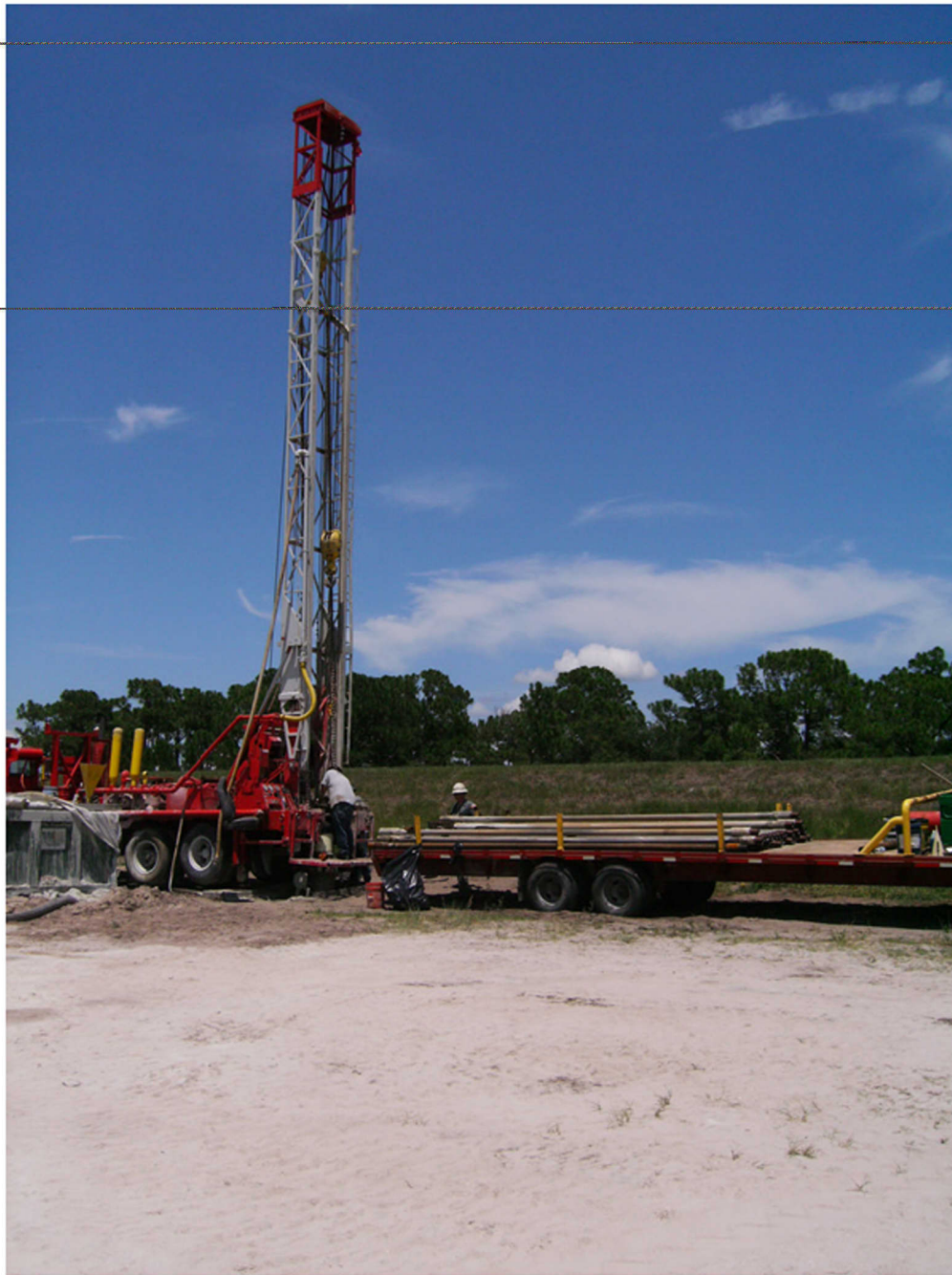
Applied Drilling Engineering drilling the 17-inch pilot hole
