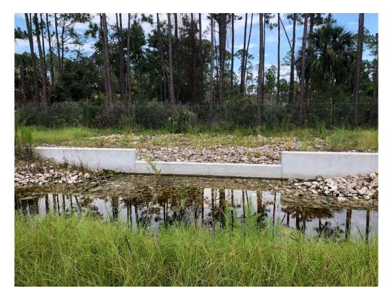
Image 12. View of concrete perimeter ditch weir.
