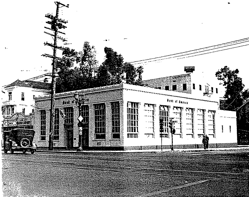
Bank of America-Echo Park Branch in 1941, 1572 W. Sunset Boulevard, (Bank of America Collection)
