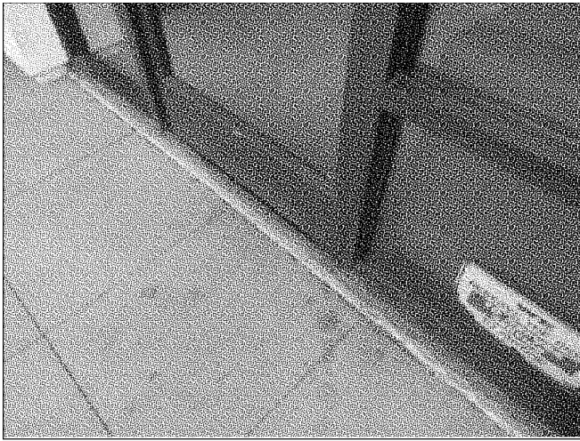
109. The threshold appears to exceed code allowable height at retail entrances
