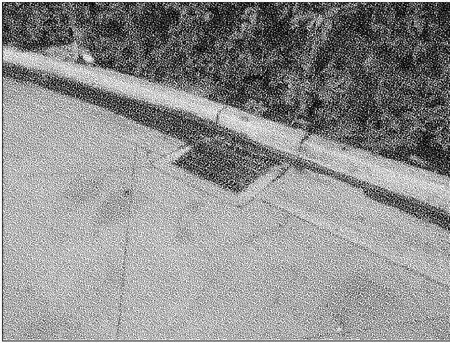
1. Curb and gutter with drain inlet
