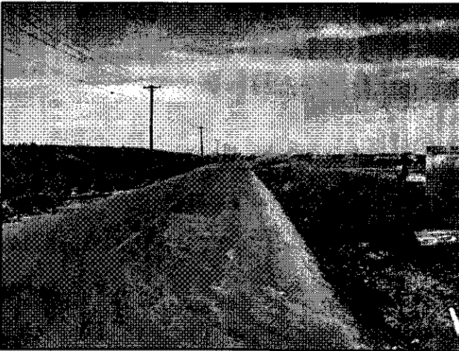
Looking west along Phillip Road
