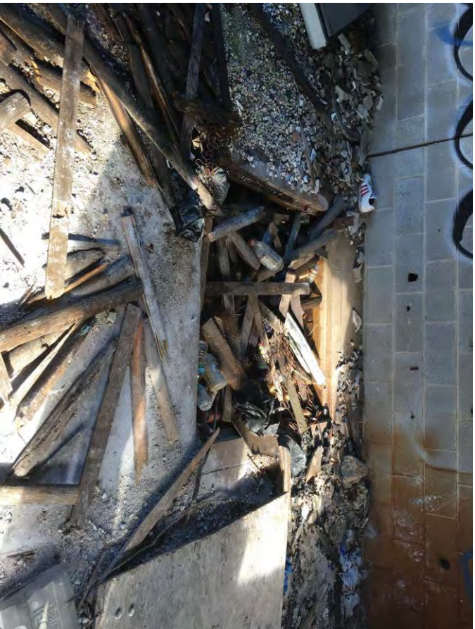
Photo 14: In-ground structures in building 5/C.
