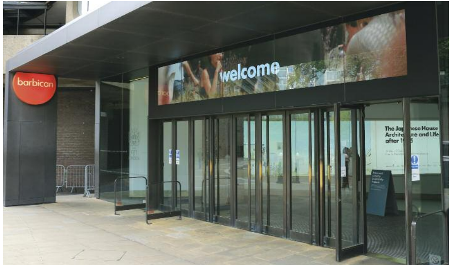
The Christie® Direct View LED screen at the main entrance of the Barbican in London.
