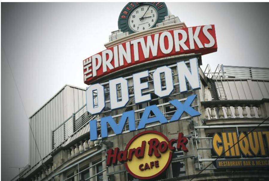
IsGroup made nine tonnes of supporting steelwork for the project.
