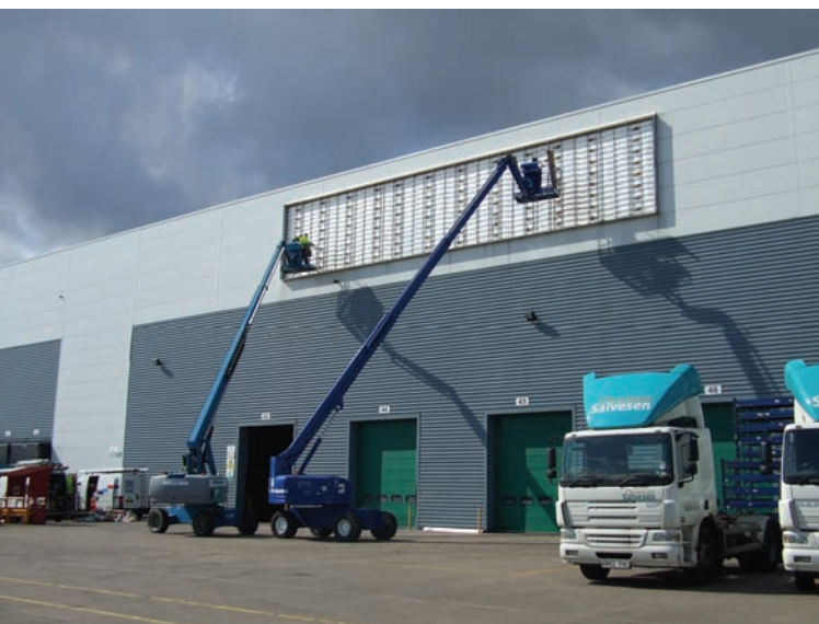
Installation by Mida Sign Services.
