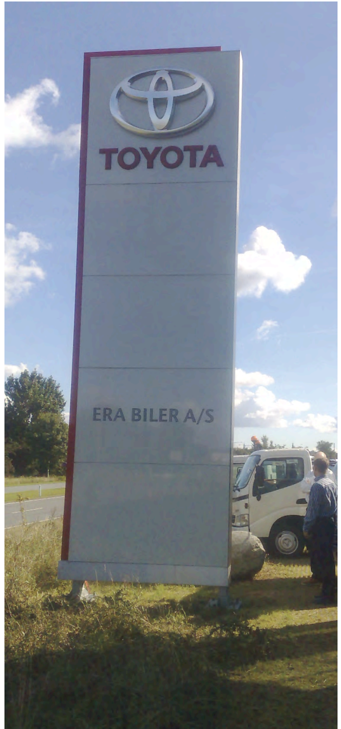
Sign erected using GroundPlug foundations.
