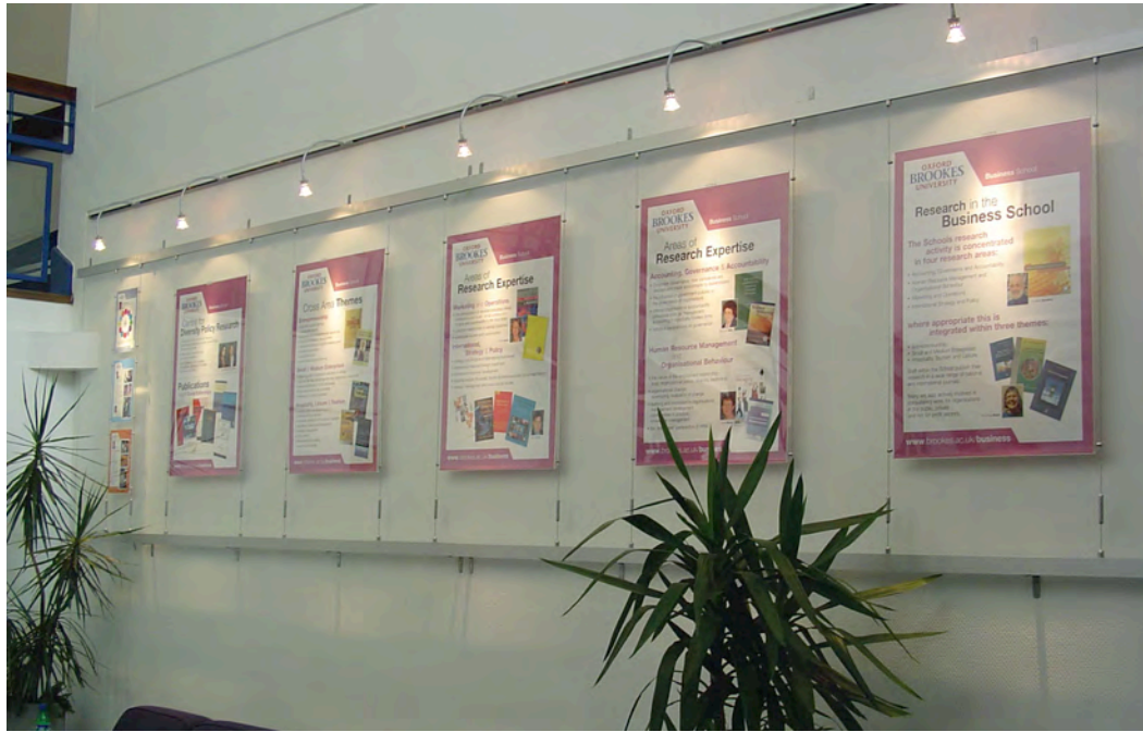
Fairfield cable system fixed between wall mounted channel with track lighting. The cables can easily be repositioned to take different size graphics.
