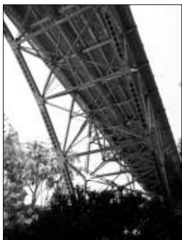
First Avenue Bridge
