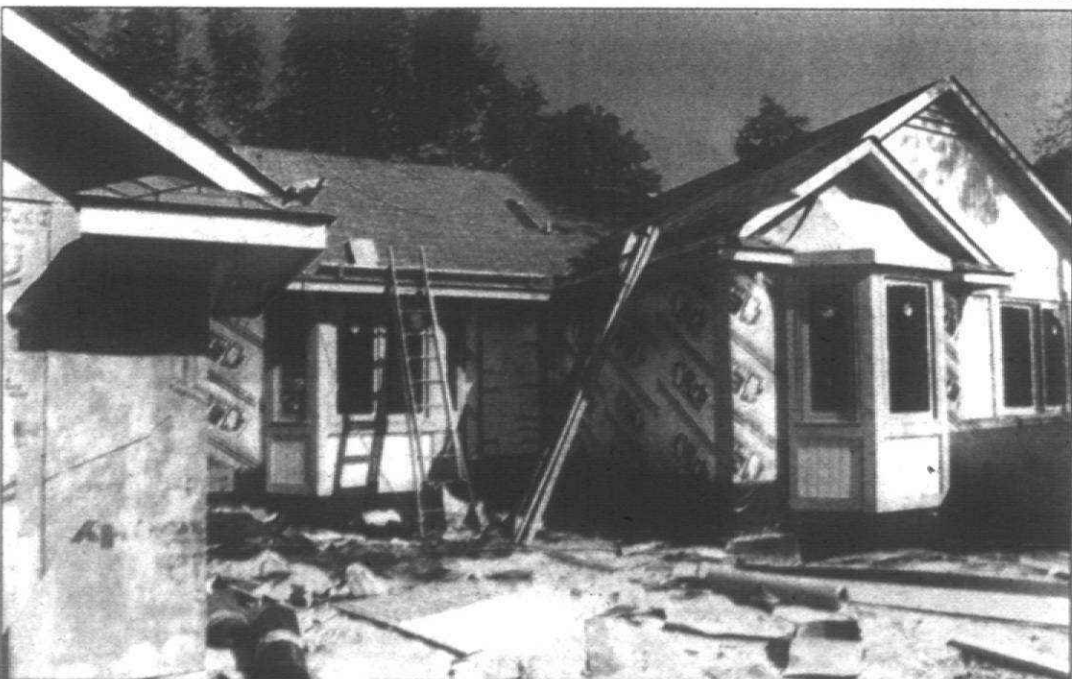
Improved insulation and windows substantially reduce heat and cooling loss.
