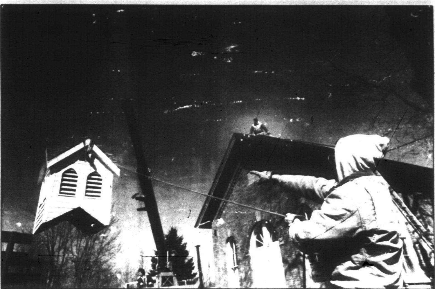
Chuck Hanlin directs the crane as the cupola is lifted.
