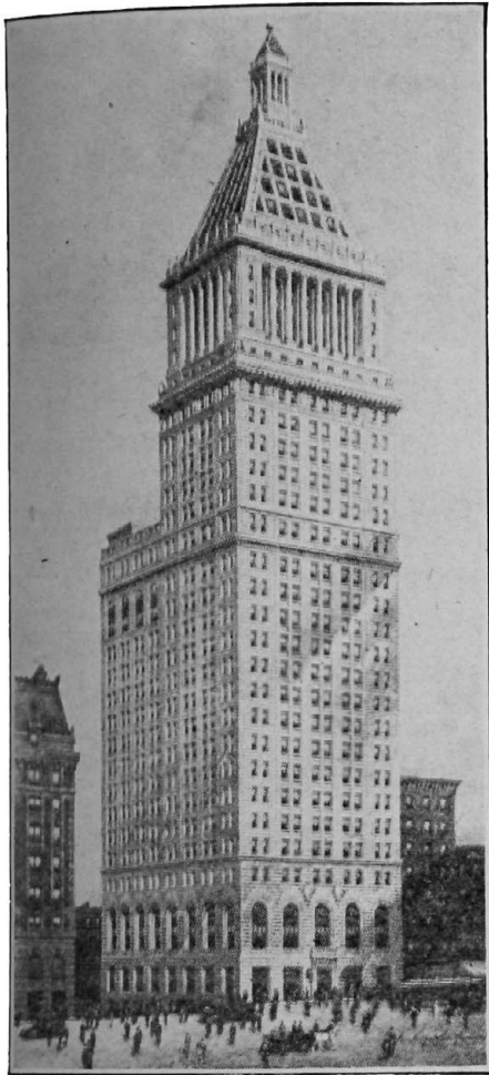
See Capt. M. W. McIntyre for offices in the Union Central Building
