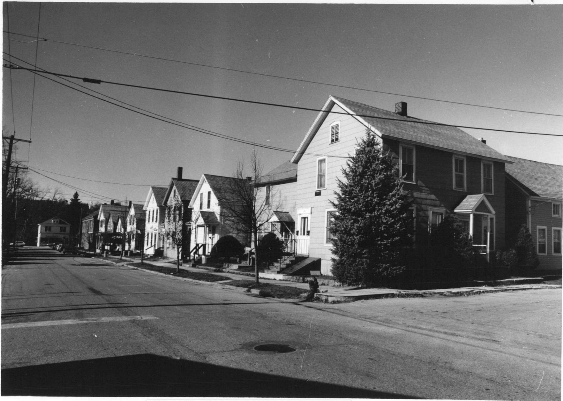
River Street streetscape NW 88-A-265 Tracy Cuning VT Division for Hist. Preservation Bennington Co. Bennington 10/88
