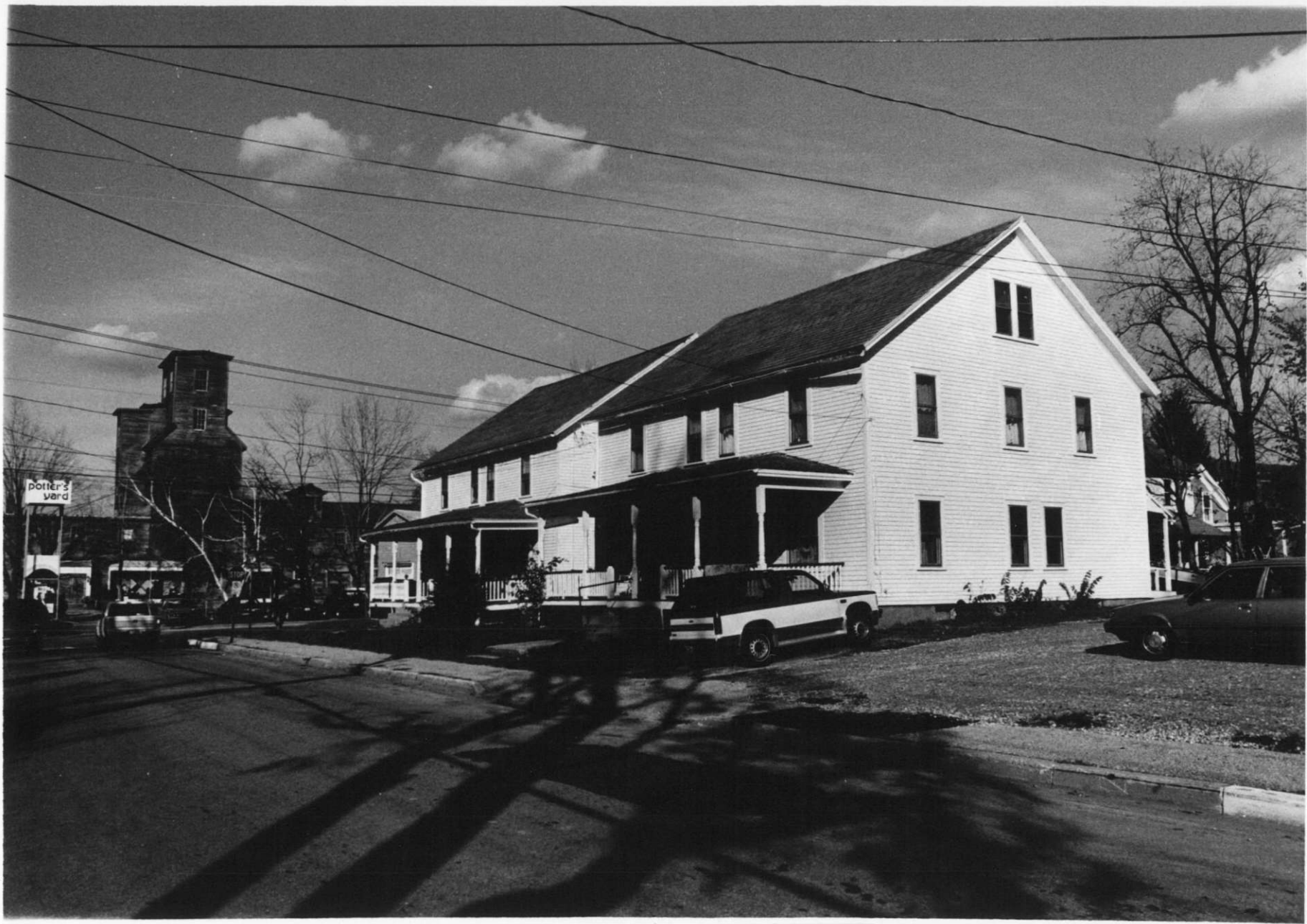
343-349 (odd) School Street NE 88-A-263 Tracy Cuning VT Division for Hist. Preservation Bennington Co. Bennington 10/88
