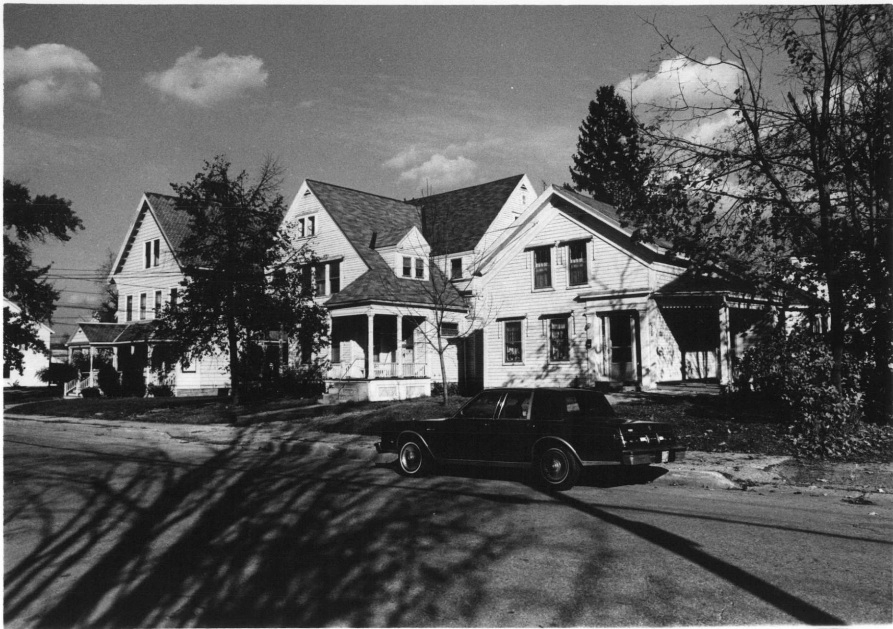
327-333 (odd) School Street NE 88-A-263 Tracy Cuning VT Division for Hist. Preservation Bennington Co. Bennington 10/88
