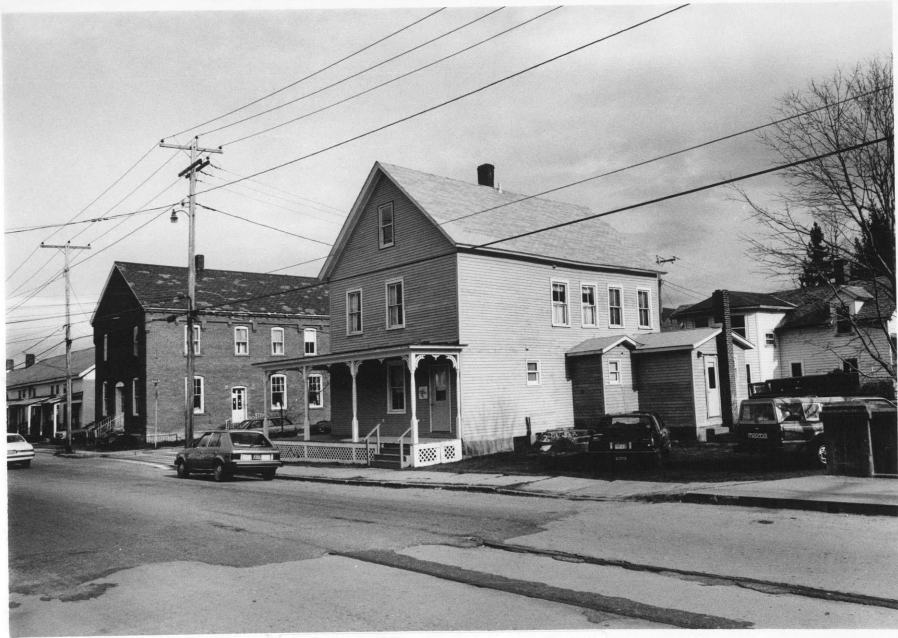
101-103 River Street NE 88-A-280 Tracy Cuning VT Division for Hist. Preservation Bennington Co. Bennington 10/88
