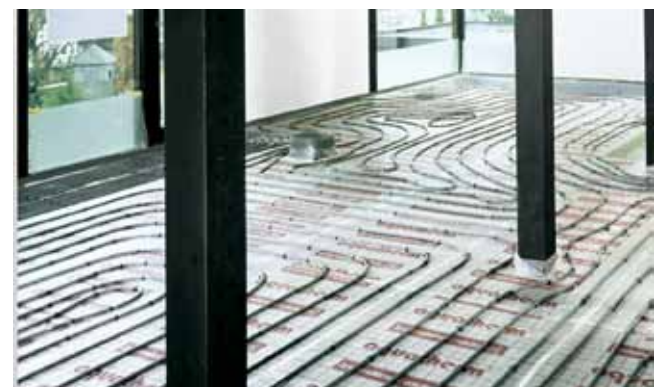
Underfloor heating installation
