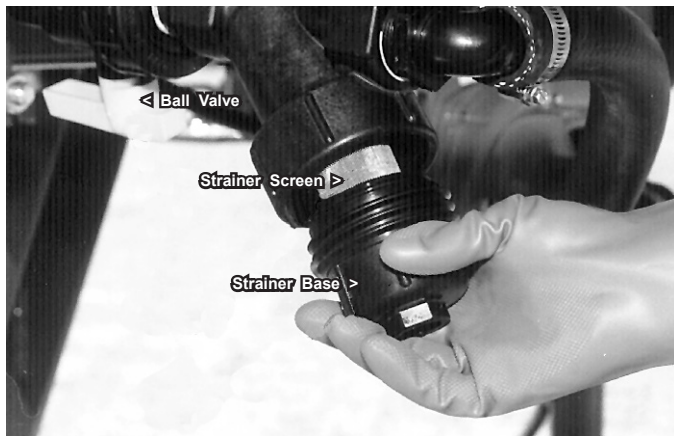
Figure C1 Removing Strainer Screen
