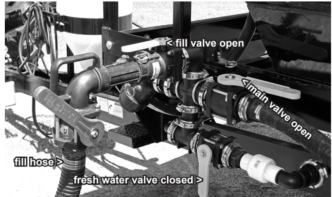
Figure B2 Filling Spray Tank
