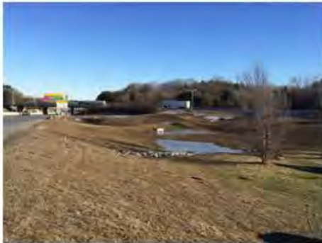
Weston Tolls – Wet Pond construction complete
