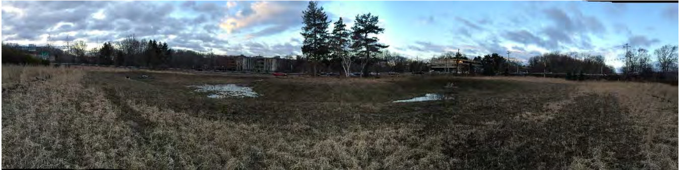
Photo 1. BMP 13, Infiltration Basin – Looking West
