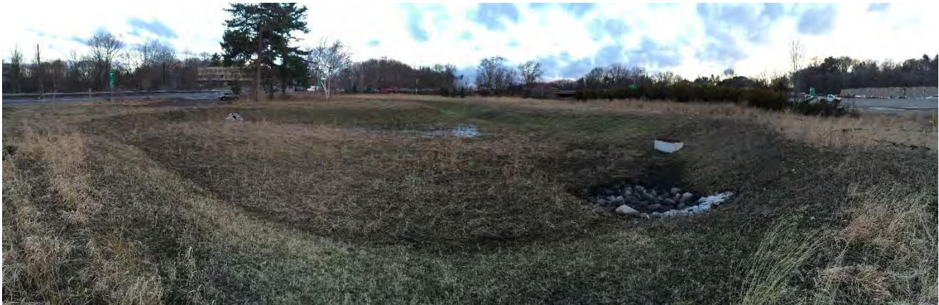
Photo 2. BMP 13, Infiltration Basin – Looking North
