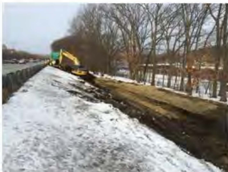
Boston- I-90 Westbound- Infiltration Basin construction
