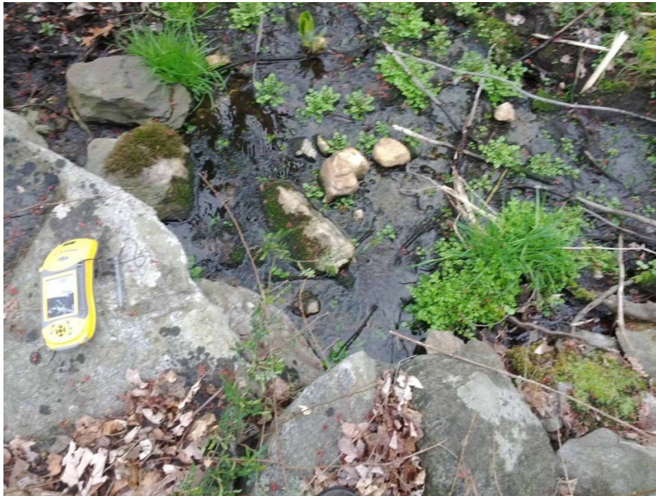
Figure 3: Discharge location below the rock retaining wall.
