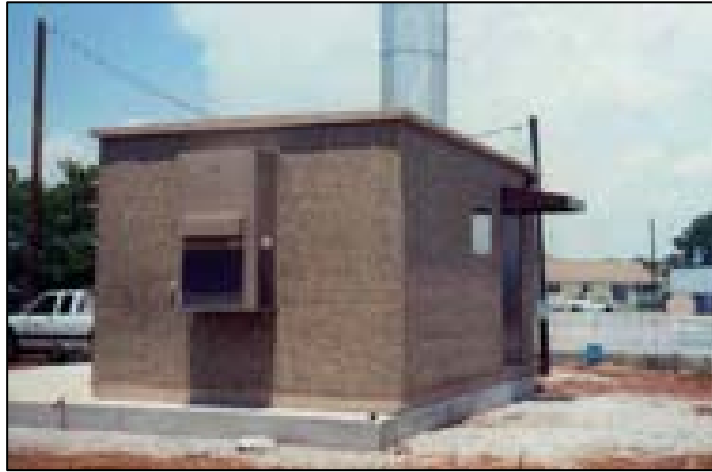
Illustration 2.2 Typical Telecommunications Hut.
