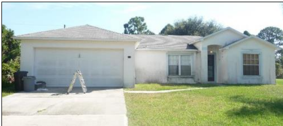
Figure 40. Site 54 prior to EIFS and window retrofits
