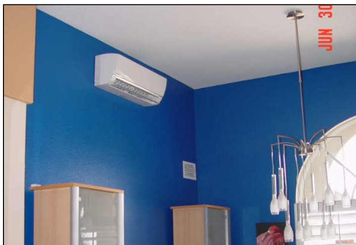
Figure ES-1. Installation of supplemental MSHP at Site 5
