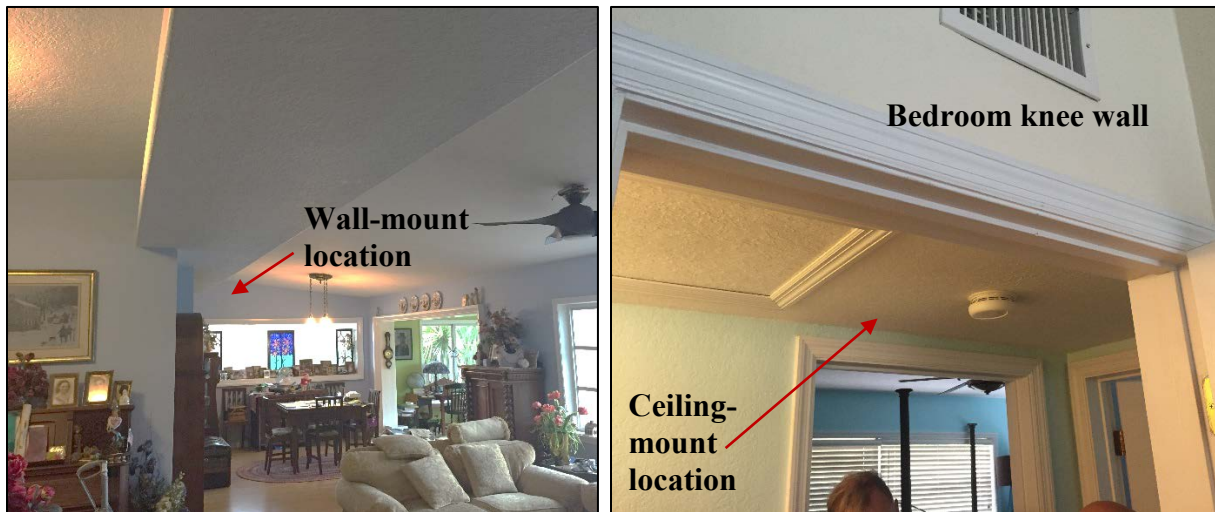
Figure 8. Chosen locations for the wall-mounted fan coil (left) and the ceiling-mounted fan coil and knee wall for supply into bedroom (right)
