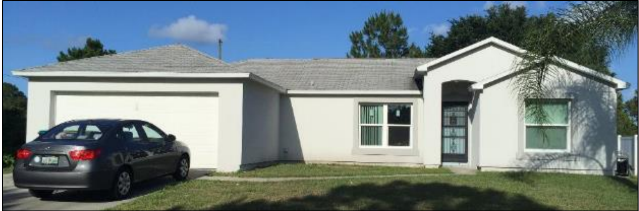
Figure 56. Site 54 after the EIFS and window retrofit
