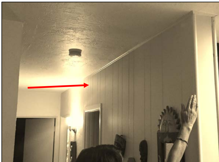
Figure 21. Ducted MSHP installation site. The arrow indicates the new fan coil location.
