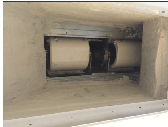
Figure 16. Air barrier applied to inside of return plenum
