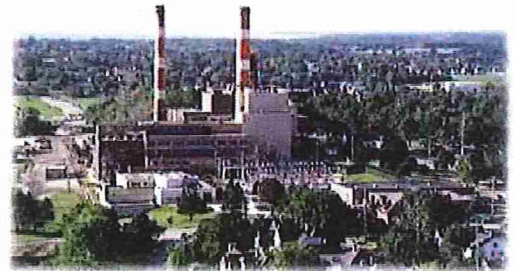
Manitowoc Public Utilities power plant in Wisconsin.
