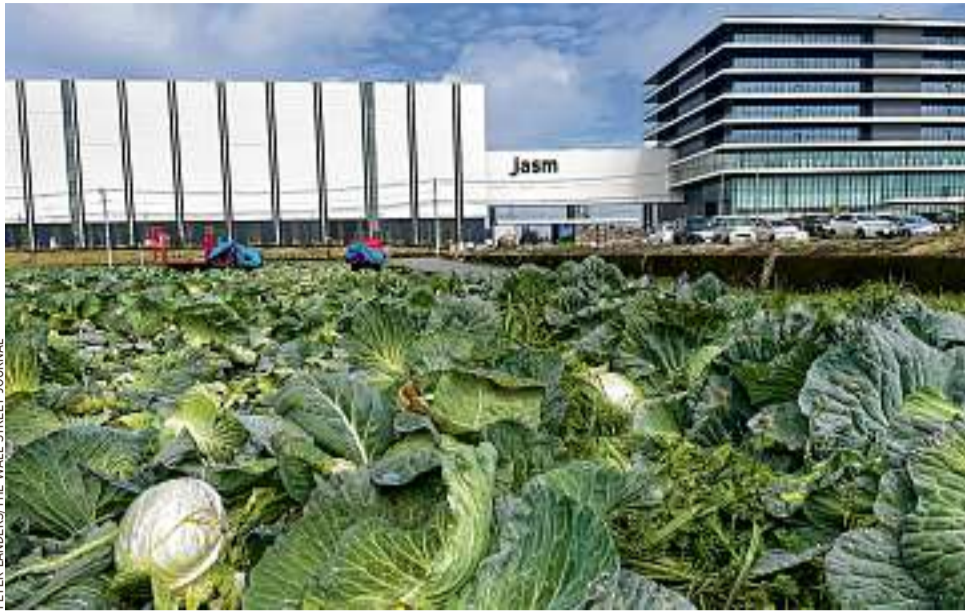
The TSMC chip factory in Japan, left, was built in less than two years. The company's Phoenix plant, which isn't identical, has faced delays and won't open this year as originally planned.
