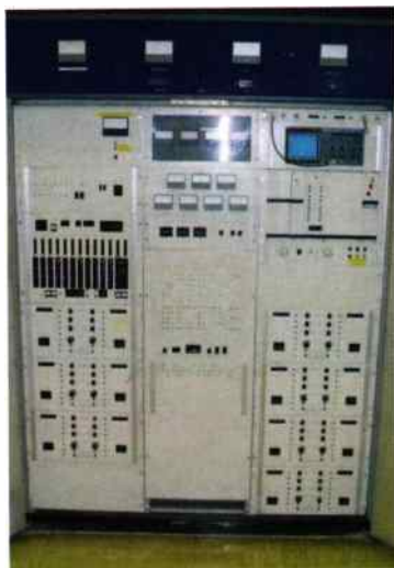
● Sender 45, a Marconi B6128 500kW a.m. transmitter.
