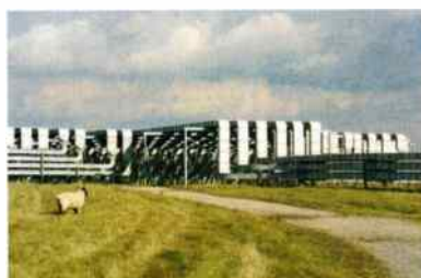
● The array baluns and switching area. Note the screened feeders running out to the arrays.
