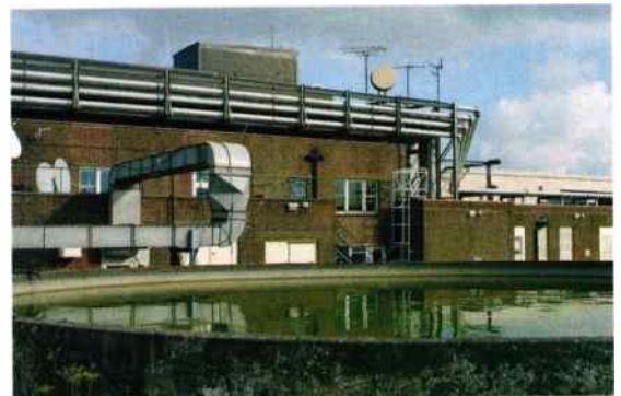
● Unlike Woofferton, the senders at Rampisham provide coaxial output. Here, behind the well stocked 'water feature', are the coaxial feeders running along the main building.
