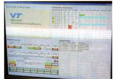
● The newly developed graphical interface to the station control system.
