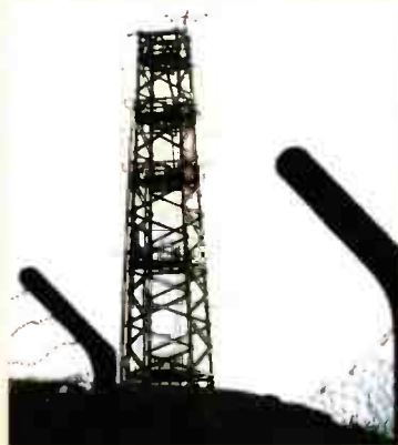
The last remaining mast in current use by the CAA. (Photograph courtesy Peter H. Goodbody, Ventnor, I.O.W.)
