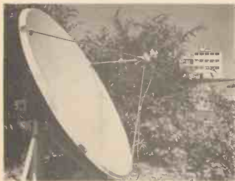
(Left) The NEC dish antenna sited in the garden and (above) the stack-mounted low noise converters.
