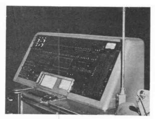
The world's first commercial data processing computer, completed in time for the 1950 U.S. Government population census. Large racks of equipment not shown in this photograph house the computer, the console being the data input and control point. (Univac)
