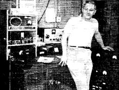
W2MEL presents a real case for "home brew" with that E.N.Y. c.w. topper of 1.2 million. On the shelves at the left is the receiver (a prototype in a constant state of change, therefore without panels). At the right is the control for switching outside antennas and exciter (v.f.o. through 2-6146s). At the extreme right is a small rack housing a pair of 813s and power supplies.
