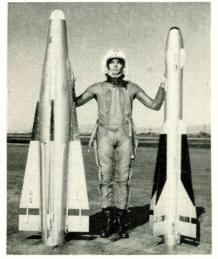
Test pilot Bart Warren holds air-to-air guided missiles, the HM-55 (1) and the HM-58 Falcons, which are being developed for the Swedish Air Force by Hughes Aircraft Co. of Culver City, Cal. Missiles will be manufactured in Sweden to Hughes' design. The HM-55 is radar guided and the HM-58 is infrared guided.
