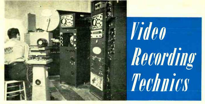
Video recording installation at Station WABD showing Eastman television recording cameras, video recording monitors and associated control equipment
