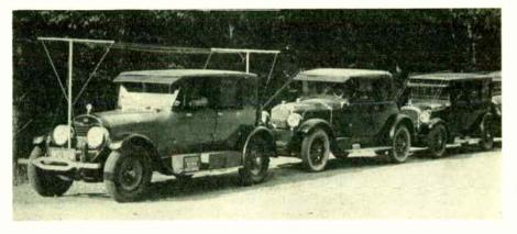
The 50-watt broadcast transmitter carried on the first car was assigned call-letters WGMU and operated on 63 meters. It was used as a remote pickup for the old Grebe station WAHG, in Richmond Hill, L. I., N. Y. Also designed by Ralph R. Batcher, author of the nostalgic article on preceding pages, was the receiving installation on Batcher's own car, second in the line, which used as antenna a four-turn loop surrounding the car.
