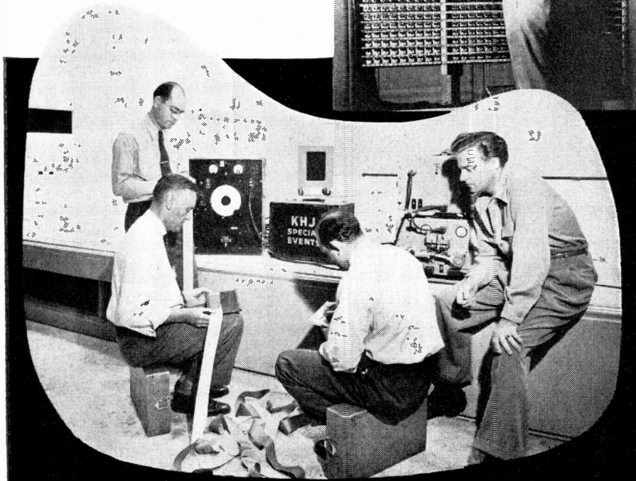
Earl Grant (left, standing), Don Lee Engineer; D. P. Loye, Technical Construction Superintendent for Western Electric; J. Garafalo, Western Electric Engineer; and Walter Carruthers, Chief Engineer, Studio Division, Don Lee, make sound measurements during construction of one of the large auditoriums.
