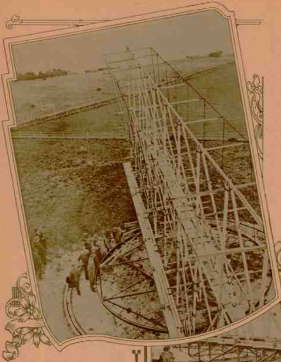
FRAMEWORK OF REVOLVING ANTENNA. This antenna is of the beam transmitter type, so that the signals will travel in as narrow a path as possible. An idea of how narrow this path is may be gained from the chart on the opposite page.
