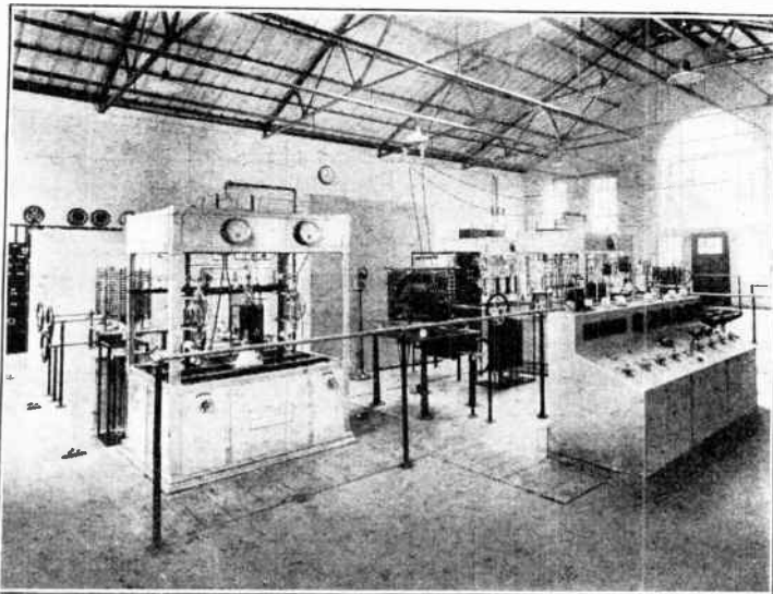
At the left is the independent drive panel, next is the coupling coil to the amplifier. In the foreground is the engineer's control panel.
