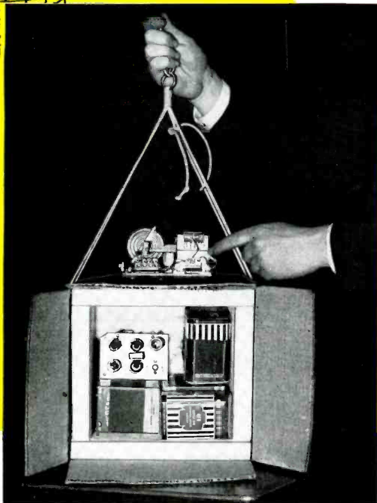
Transmitter ready for flight. Atop box is a registering aneroid barometer.
