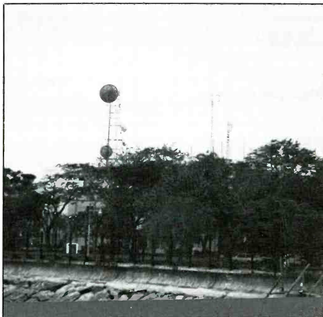
Another view of the embassy compound as seen from Manila Bay.
