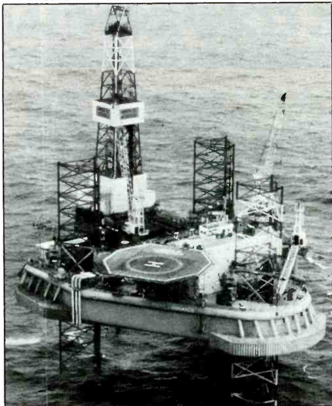
Fig. 3 - Drilling platform "Key Largo" is similar to the one shown in this picture.
